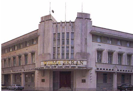
Figure 2. Anglo-Oriental Building (Source: Chen (1998), p101)
